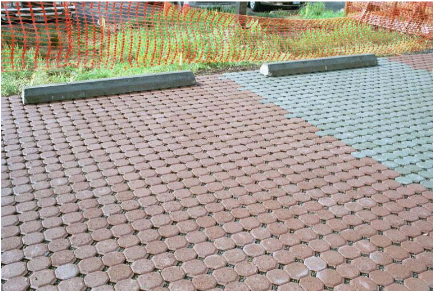
Pervious paver block (Uni Eco-Stone) parking lot at Multnomah Arts Center (SW 31 st & Capitol Hwy)
