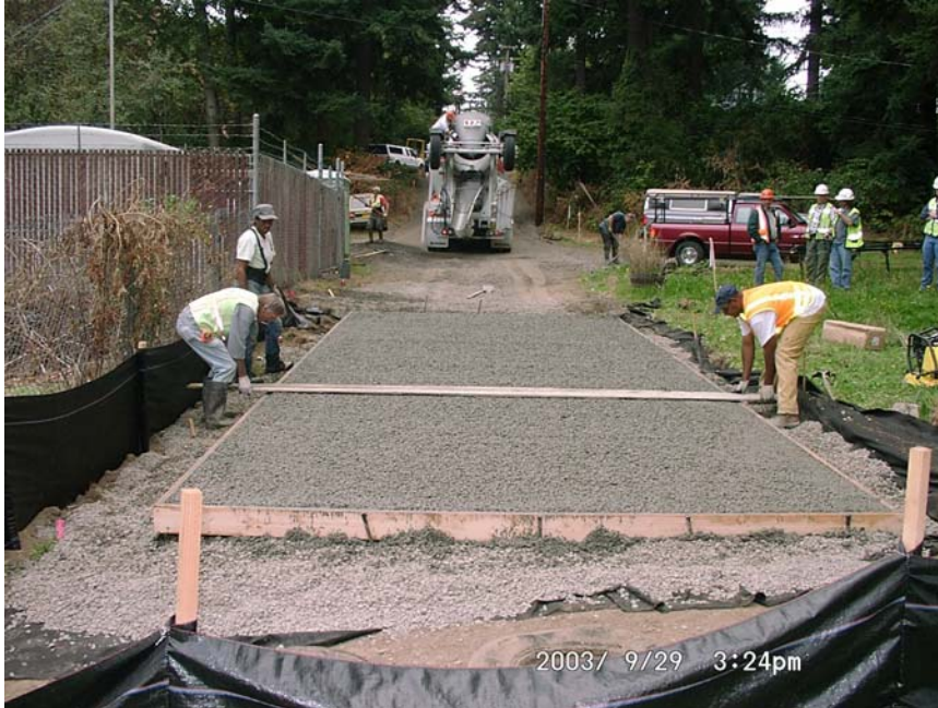
Installation of pervious concrete at NE 94 th & Broadway pump station site.
