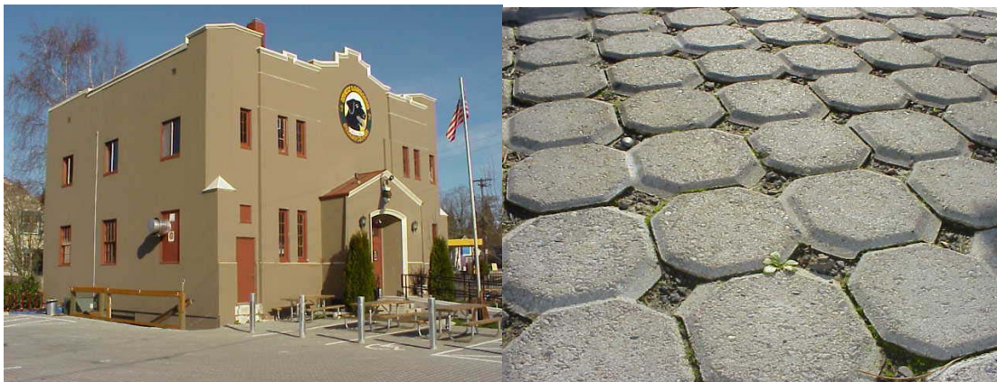
Pervious paver block (Uni Eco-Stone) parking lot at Lucky Lab Brew Pub in SW Portland (SW 31 st & Capitol Hwy)
