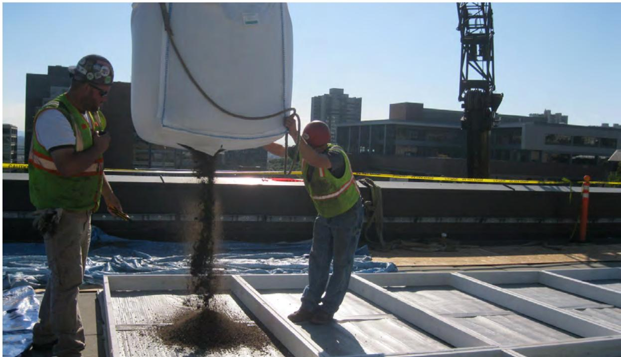
Figure 6, Intensive A-3 mixture being dumped into box B-4 (first three sections).
