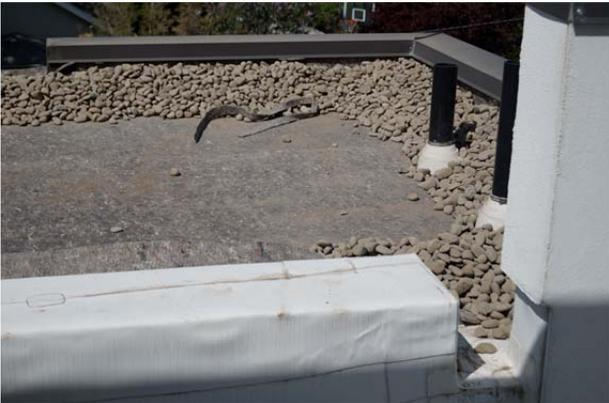
River rock, over felt liner, around perimeter of roof
