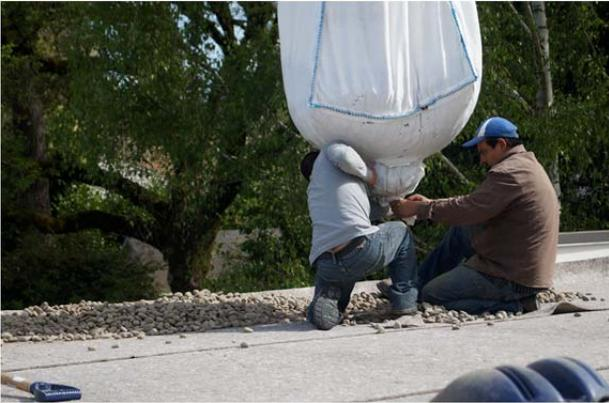
1" river rock being distributed around perimeter for drainage
