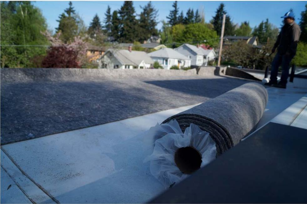
Membrane still visible, felt liner being installed.
