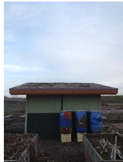
Finished Shed ecoroof.
