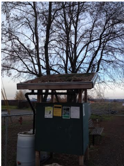
Finished Kiosk ecoroof.
