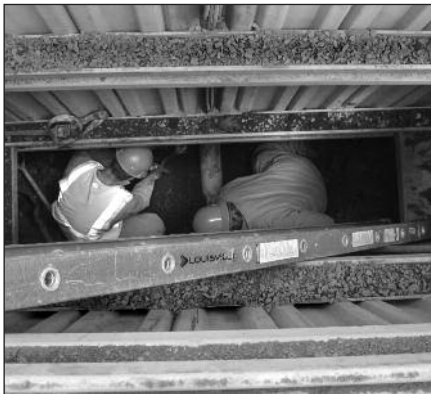
working on a lateral in the right-of-way
