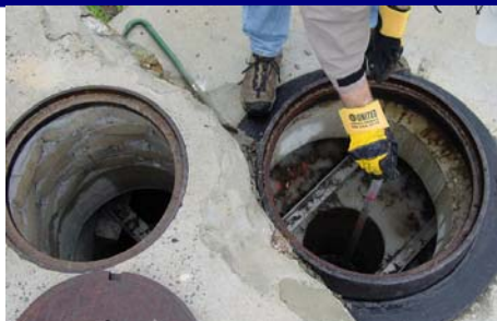
Figure 4 – Checking Sediment using a Probe
