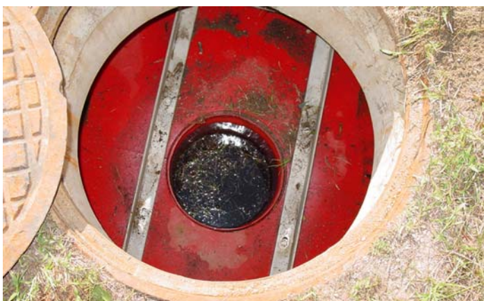
Figure 6: View over Center Shaft into sediment storage Zone
