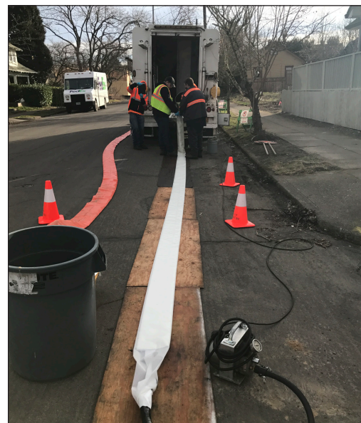
CIPP liner is prepared for use.
