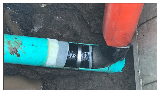
Liner is inserted into lateral.
