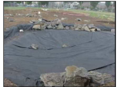
Laying the liner for the permanent pond; 2002
