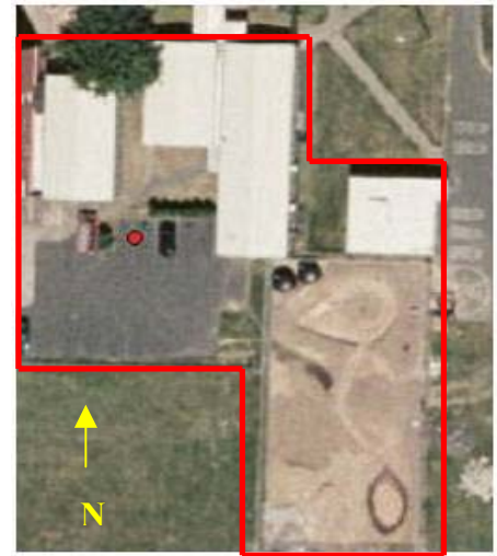
Excavation of the project in 2002. Note the outlines of the stormwater features (SE corner) and the catchment areas (adjacent classrooms and parking lot).
