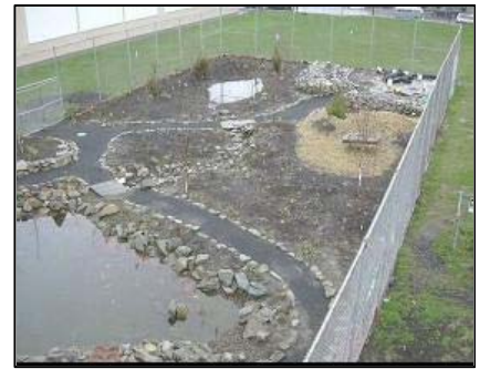
Just after construction - note landscape infiltration basin in background; January 2003
