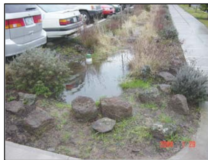
Ponding in the last compartment of the swale in winter - note standpipe
