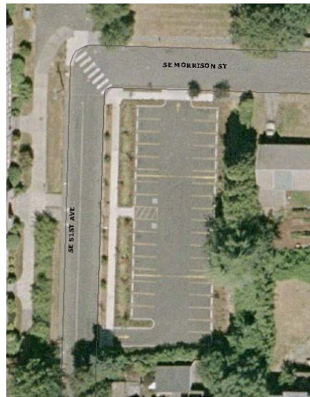
Aerial view of the same parking lot after the retrofit; 2003
