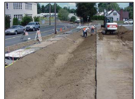
Grading the swale; August 2002
