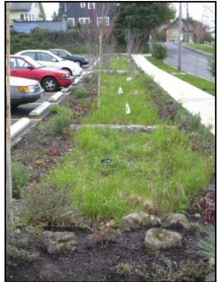
Parking lot following construction and planting, October 2002.
