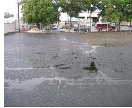
Repaved asphalt parking lot, graded to drain into infiltration basin; 2002
