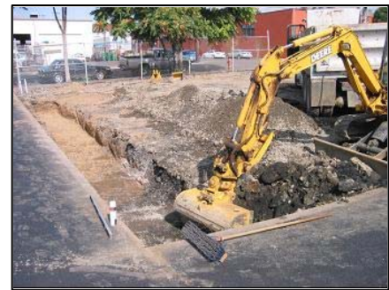
L-shaped basin under construction, 2002
