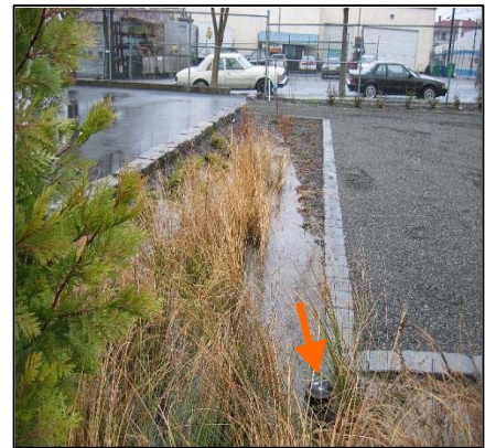
L-shaped infiltration basin with emergency overflow ( see arrow) and gravel courtyard
