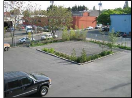
Overview of the retrofitted parking lot
