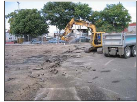
Removal of parking lot asphalt during project construction, summer 2002
