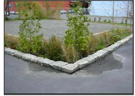
Landscape infiltration basin after a storm, 2003. Note damp pavement where runoff recently ponded on asphalt surface.
