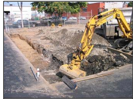
L-shaped basin under construction, 2002
