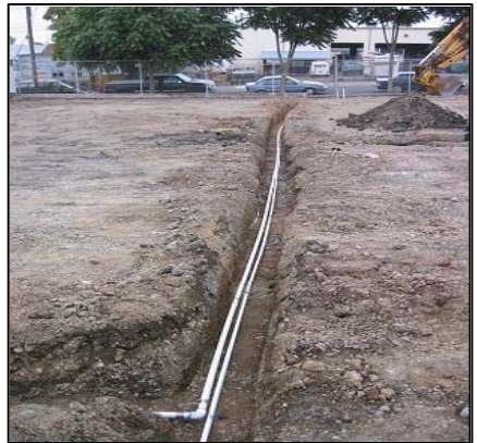
New subsurface irrigation pipe for hose bib, looking north.
