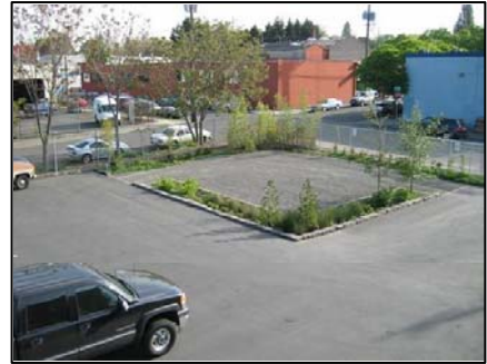
Overview of the retrofitted parking lot
