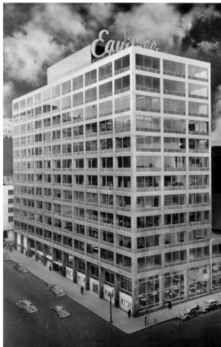
Equitable Building, Pietro Belluschi, 1948.
