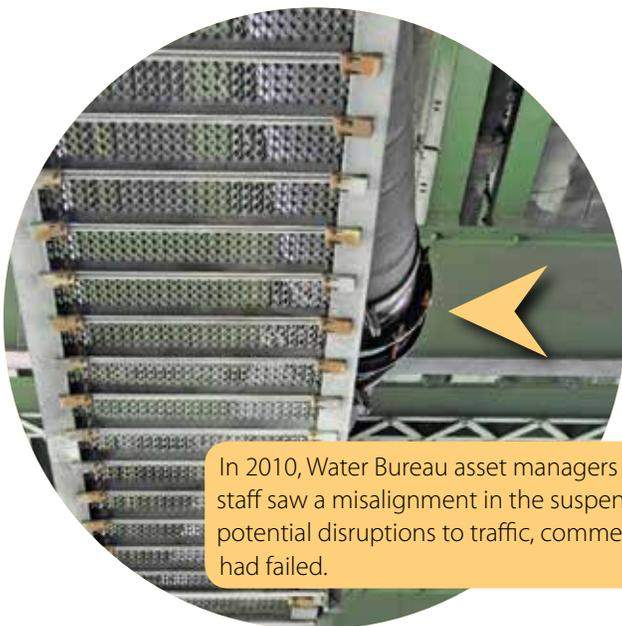
In 2010, Water Bureau asset managers inspected some of its pipes on bridges. Under the NE Grand Avenue bridge, staff saw a misalignment in the suspended water main. Repairs cost \$200,000—but avoided millions of dollars in potential disruptions to traffic, commerce, emergency response, and in repairs to the I-84 highway below if the pipe had failed.
