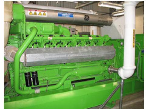
*These engine generators use biogas to produce about 40 percent of the CBWTP's electricity needs.*
