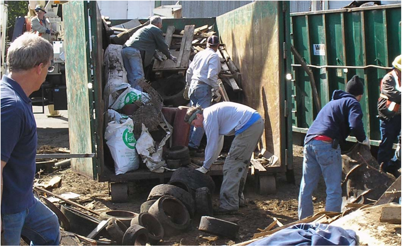
SOLV IT volunteers roll up their sleeves and help clean up site in North Portland.
