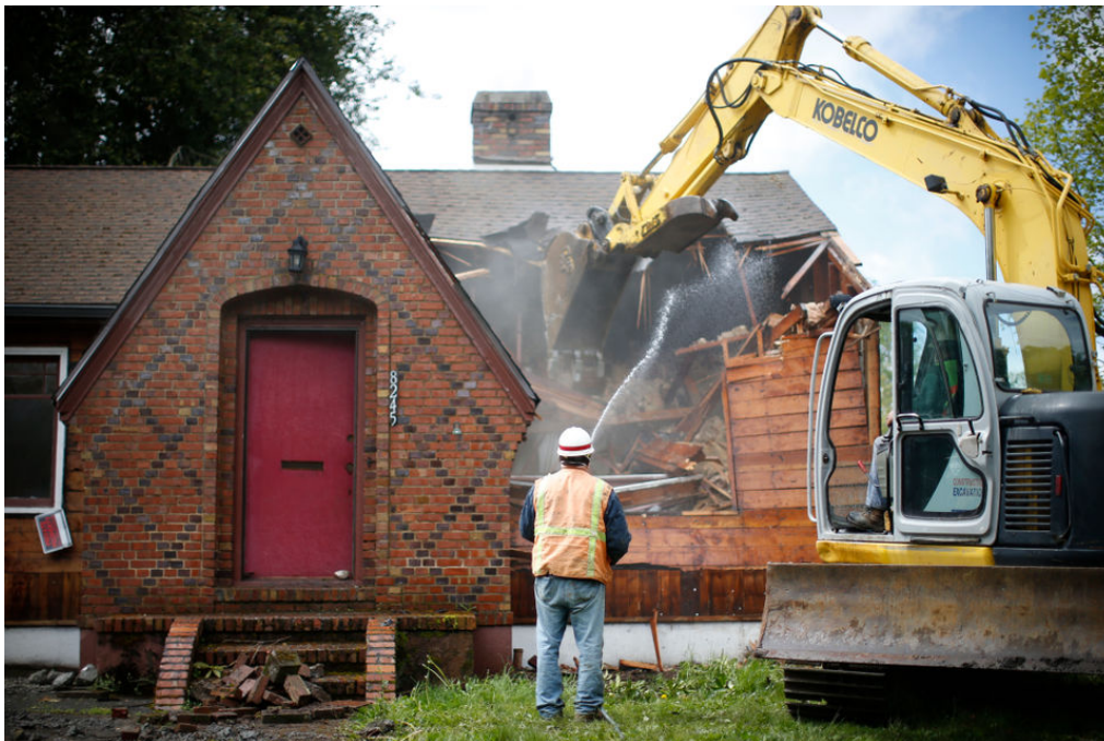
A house in the North Portland neighborhood of Portsmouth is demolished on April 26, 2017. Neighbors worked extensively with the developer, the city, the Environmental Protection Agency and other groups to ensure safe removal of the asbestos siding on the house. New city rules would require their removal by hand, as well as water misting to contain dust. (Beth Nakamura/Staff)
