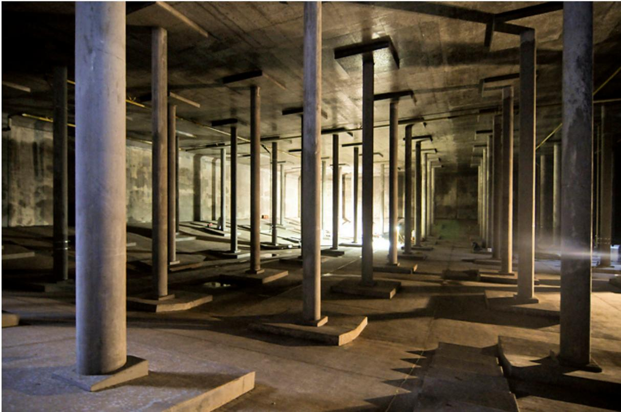
The reservoir is comprised of two cells, each with a 12.5 million gallon capacity. Both cells together measure approximately 400 by 300 feet, with a total of 252 support columns.
