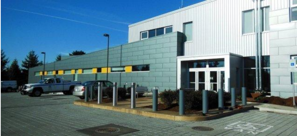
The new Emergency Coordination Center (ECC) building
