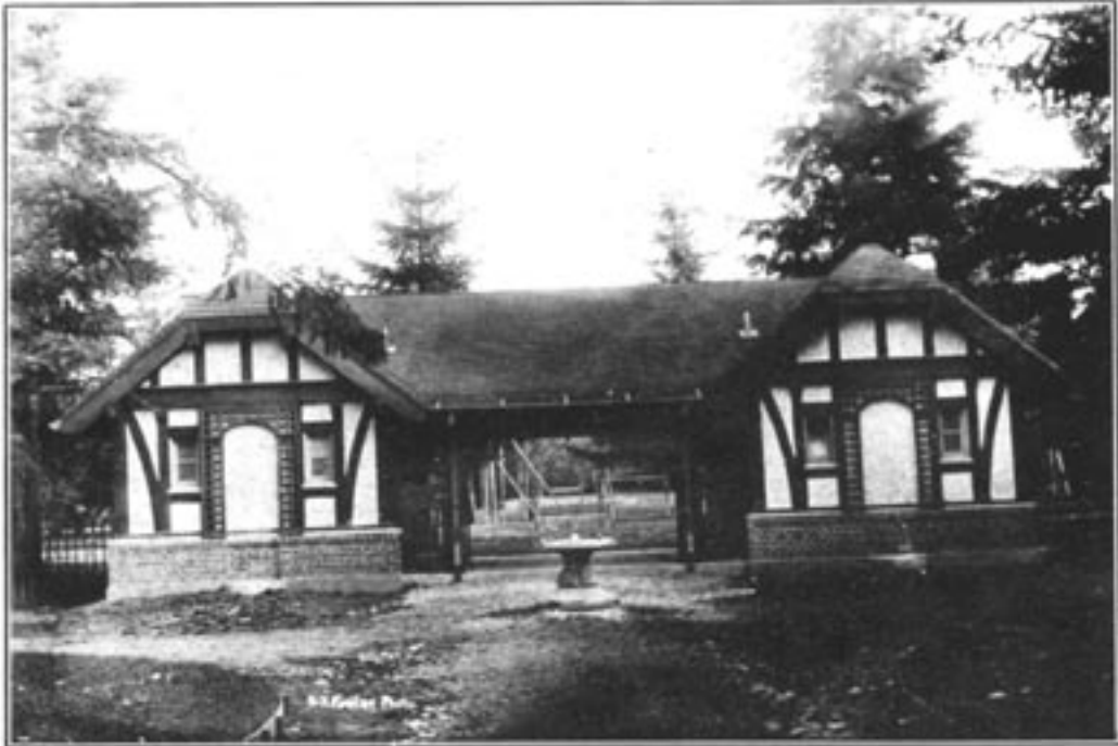
Comfort Station at Columbia Park 1912
