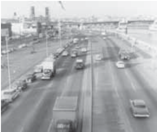
Top : The seawall under construction, 1929. Bottom : Six-lane Harbor Drive at the river's edge, 1958.
