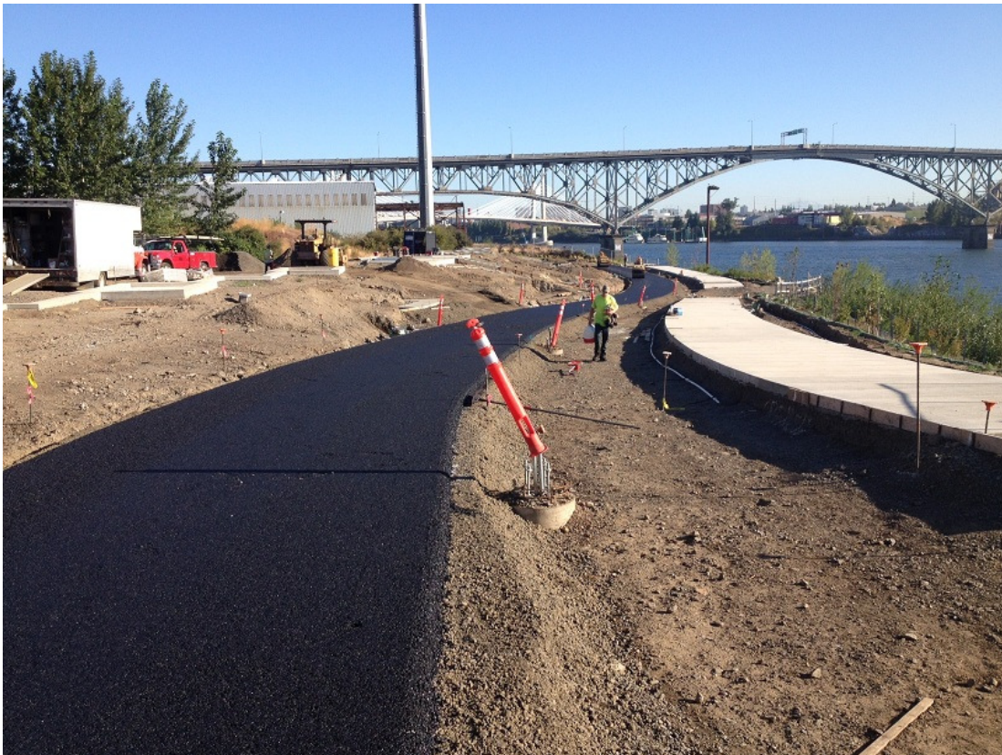
Looking north from near Curry Street. L-to-R: the concrete Upper Terraces, then the asphalt bike path, the concrete pedestrian path, and the riparian vegetation growing on the reconstructed riverbank.
