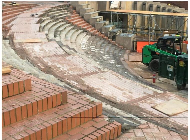
The waterproofing membrane that was underneath the bricks is also being removed. This work will continue into the next couple months.
