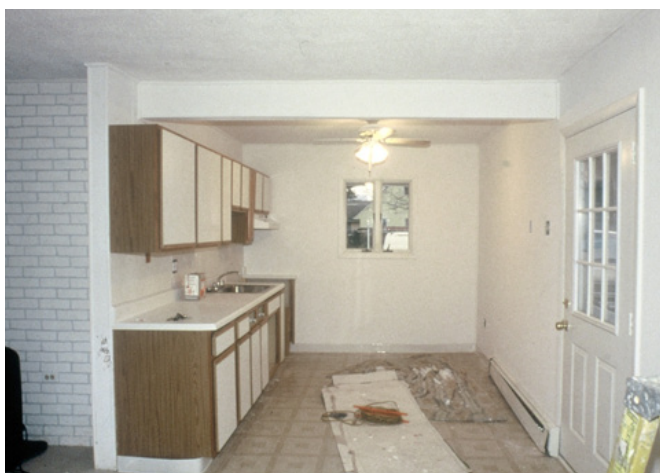
FIGURE 6.5 Unit turnover is an excellent time to conduct the visual assessment and perform lead-safe maintenance activities.
