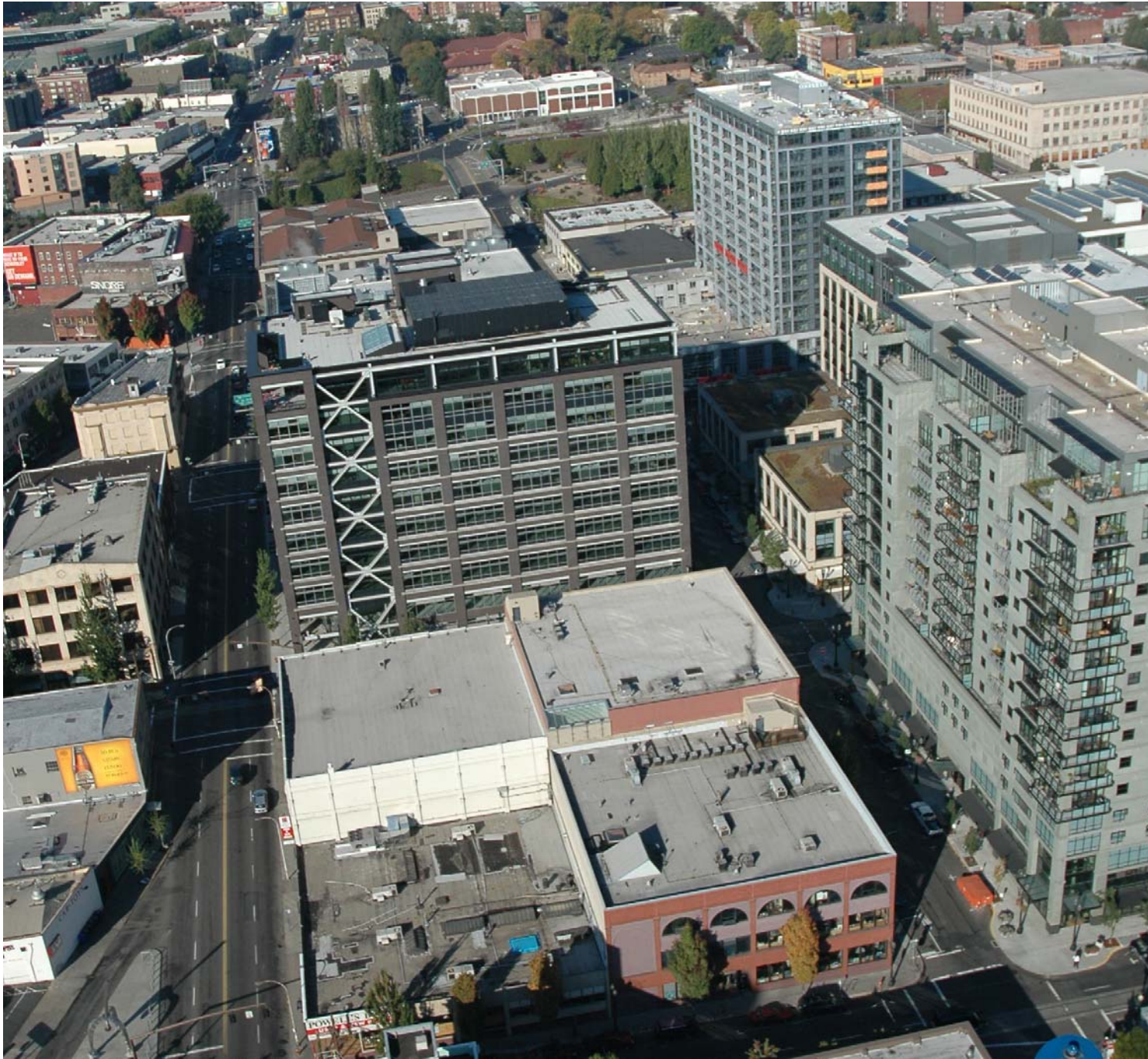
Burnside and Couch from NW 10 th Avenue west to I-405.
