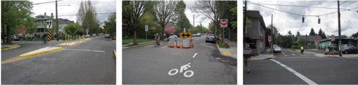
Traffic diverters are traffic calming devices that restrict certain turn movements in order to discourage a street’s use as a "cut-through" by non-local traffic.
