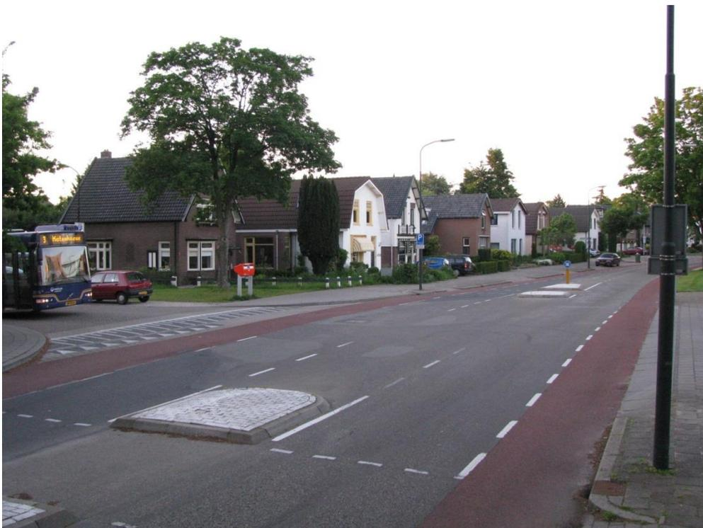
**Figure 2** Example of a reddish coloured bicycle lane for through cyclists; exit constructions at minor roads; raised middle islands that enclose a left-turn section for both cars and cyclists crossing the two-lane priority road.
