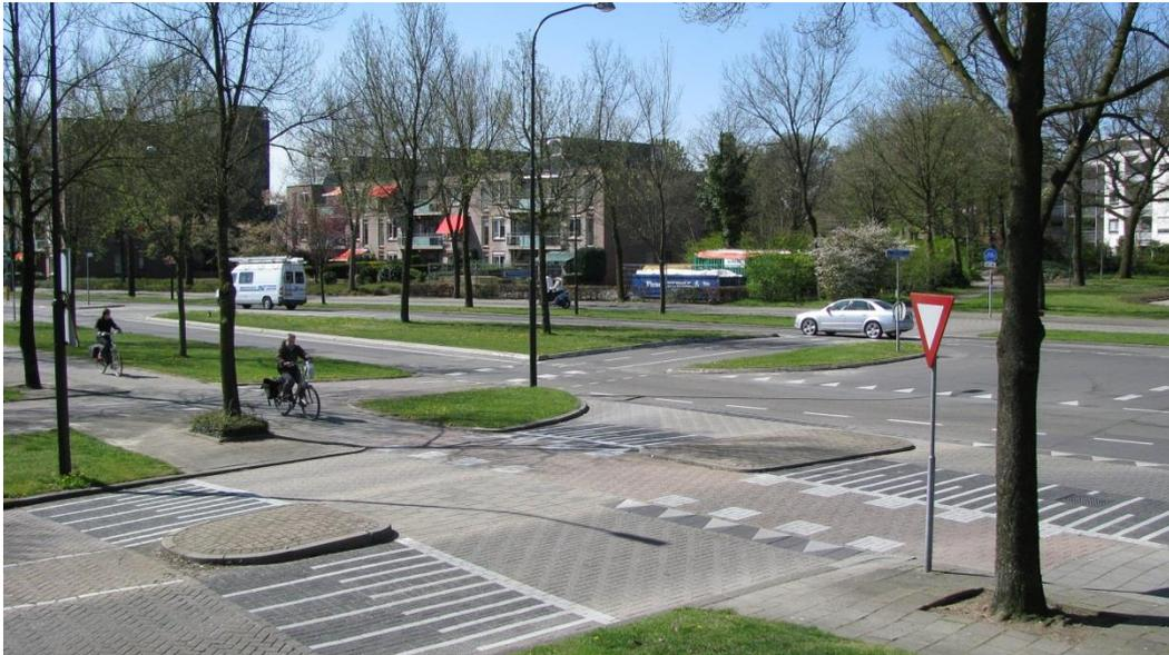
**Figure 1** Example of a well-marked, reddish coloured, raised bicycle crossing for through cyclists on a one-way cycle track with a distance of over five meters from the priority road; a raised middle island with a separate space for cyclists crossing the two-lane priority road.
