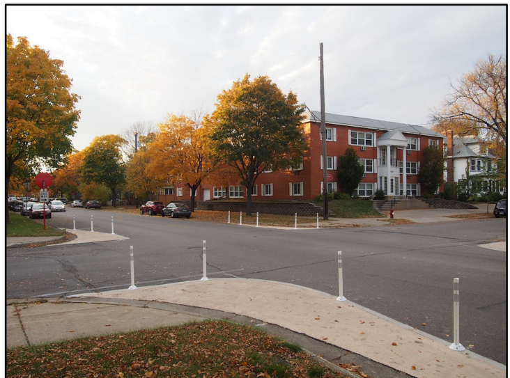
Paint & post curb extensions in Minneapolis
