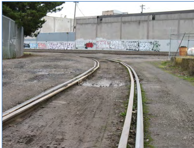
Figure 2: Muddy condition of Southerly Lead
