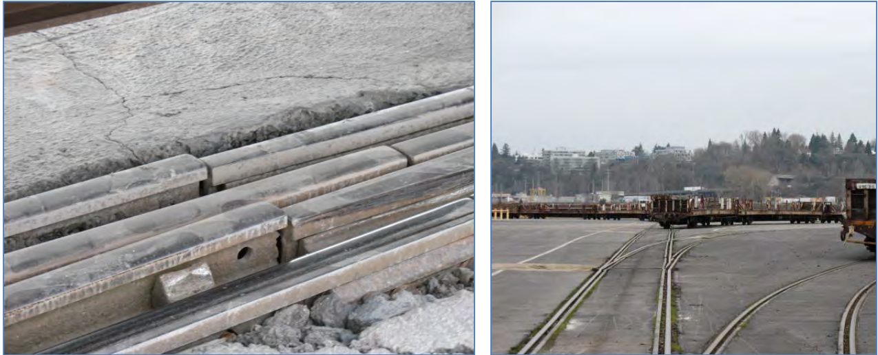
Figure 3: Left: Typical view of turnouts showing joint pounding, mis-aligned guard rail, etc. Right: Looking up the switch ladder towards the berths.
