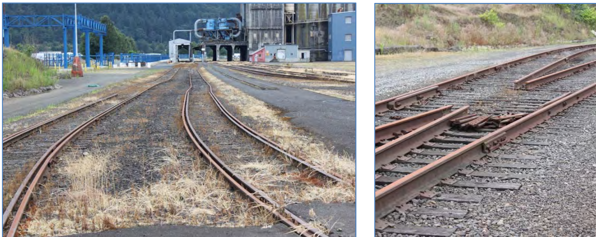
Figure 9: Left: View of Tracks 708 & 709. Right: Missing switch frog at west end of Tracks 708 & 709.
