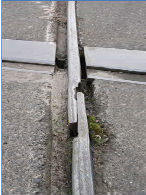
Figure 4: Rail expansion joint showing head flattening and chipping.
