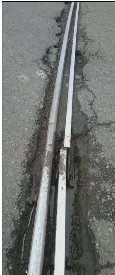
Figure 7: Mis-aligned and loose rail in crossing.
