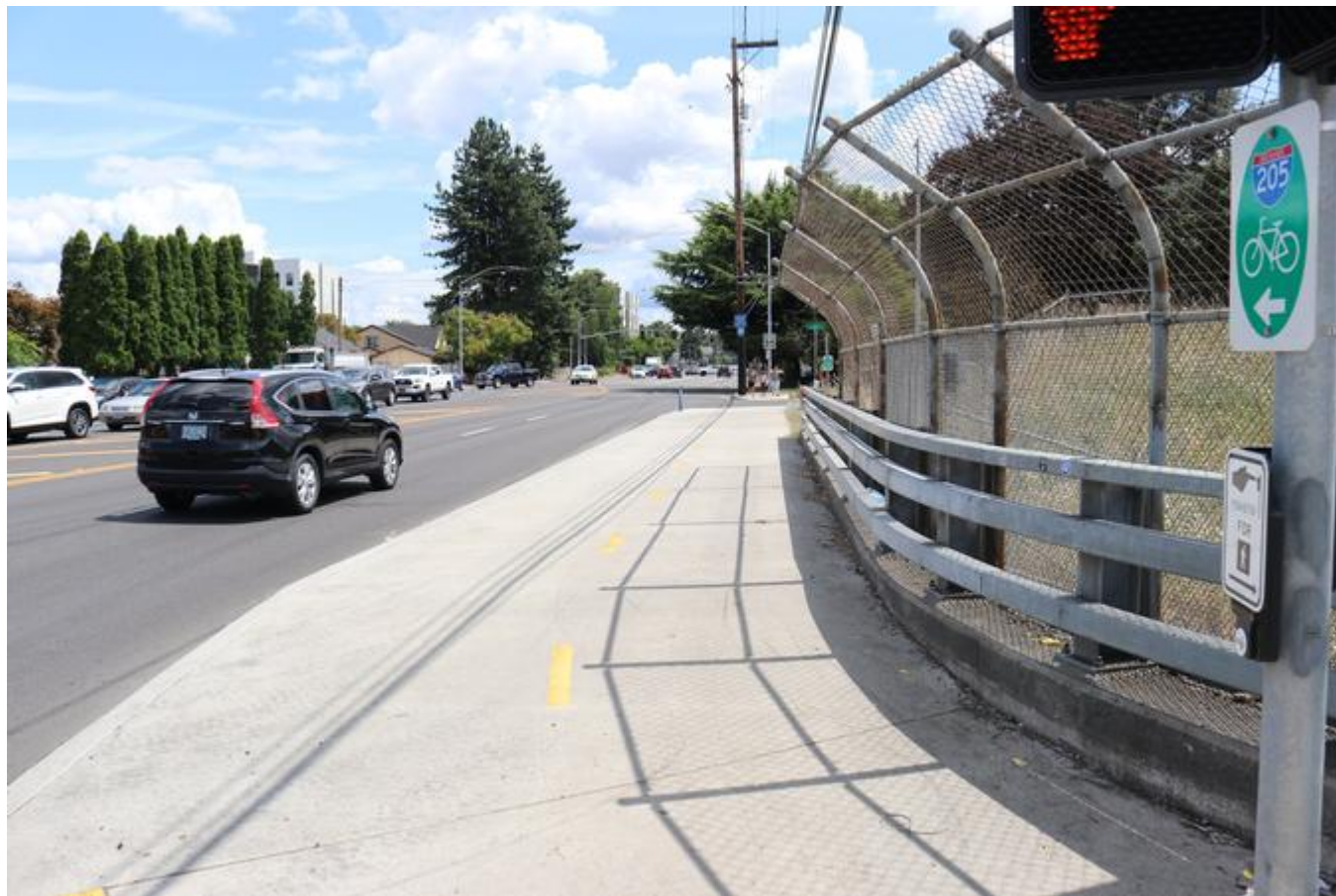
A 2018 partnership between PBOT and ODOT provided a safer crossing of NE Glisan Street at the I-205 Multi-Use Path, including wider sidewalks, larger curb ramps, and upgraded signals.
