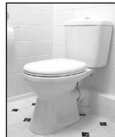
To check your toilet for leaks, lift off the toilet tank lid. Without flushing, place 1 dye tablet (or 10 drops of food coloring) in the toilet tank. Wait at least 15 minutes and check the bowl of the toilet. If there is dye in the bowl, the toilet has a leak.
