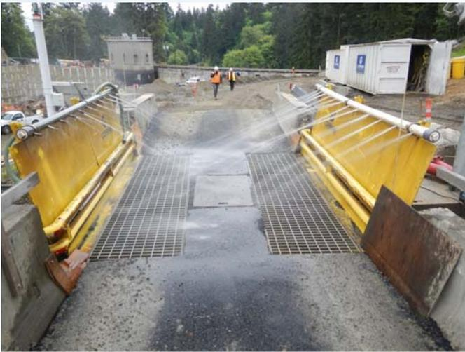
Crews installed a wheel wash to help keep dirt, gravel and other materials on-site and off roads.
