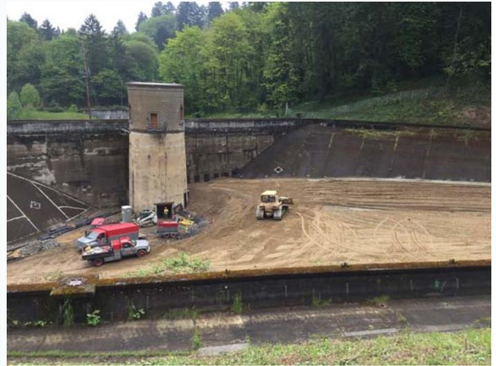
Above photo shows lower reservoir site in May 2017, and below shows May 2018. Over the past year a lot of material has been moved onto the site, much of it coming from the excavation in the upper reservoir site. This is in preparation for the new lowland habitat that is being built on this site.
