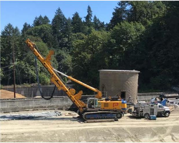
Drilling rig assembled and ready to start drilling 176 shafts, some of them up to 100 feet deep.
