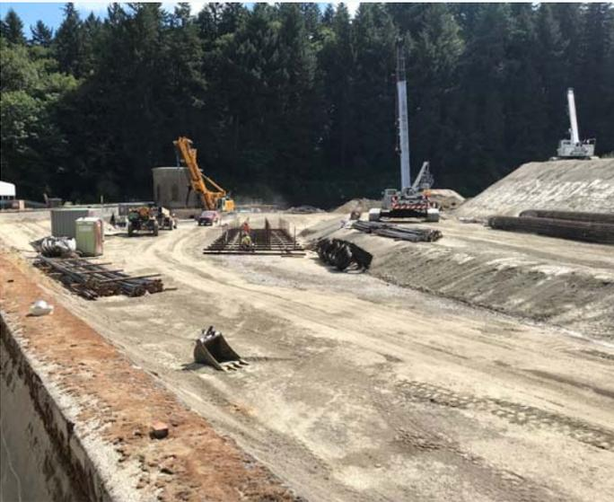
The lower reservoir is being used as a fabrication site to assemble equipment and build rebar cages. Rebar cages will re-enforce the 176 drilled shafts.
