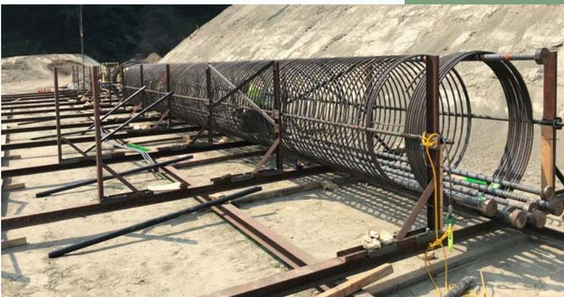
The rebar cages (pictured to the left) are constructed by crews above ground and then lowered into the drilled shaft. Once in place concrete is poured to fill the shaft with the rebar cage providing reinforcement. Each rebar cage is built to the length needed for a particular shaft.
