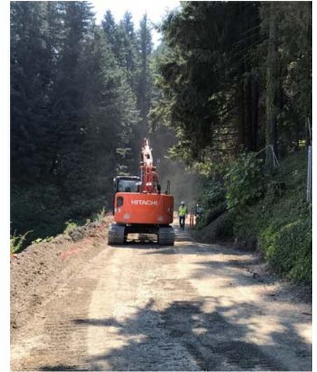
A crew had to widen Murray Road in preparation to move a crane from the lower reservoir area up to the new reservoir site. The crane has a top speed of .9 miles per hour. It will take more than 8 hours to move it into the new location. Once there, it will assist in the off loading of the tower crane and its assembly on-site.
