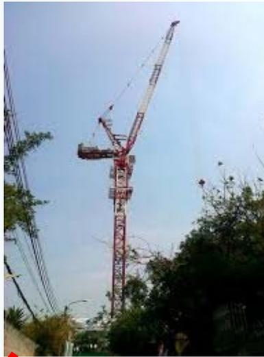
Pictured above is a luffing boom crane, the type that will be erected on-site this month. This type of crane was chosen for this site because the boom can be moved, stowed and operated while extended or in an upward direction. This allows the operator to avoid the surrounding trees.
