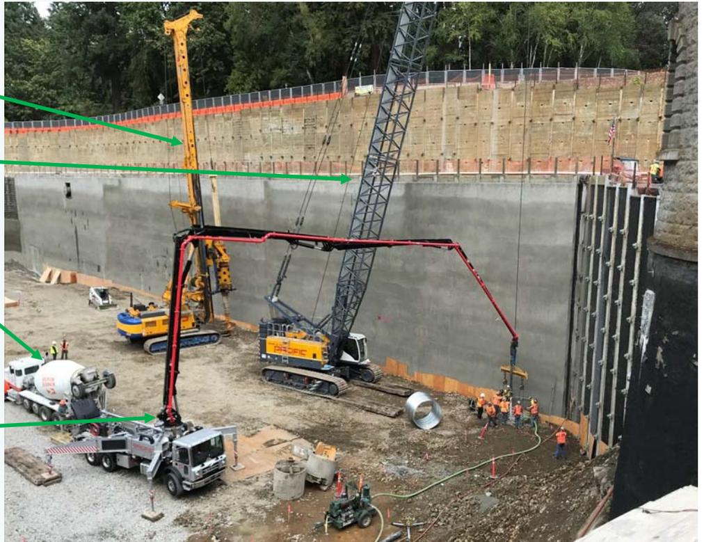
Concrete being pumped into the shaft.
