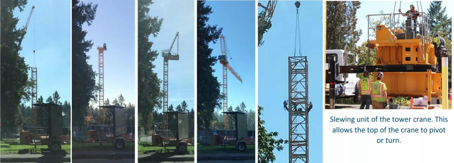
Slewing unit of the tower crane. This allows the top of the crane to pivot or turn.
