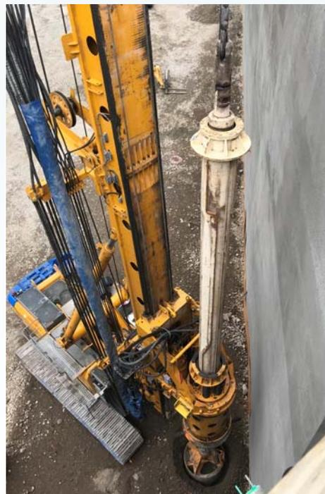
Right: The drill bit being used to drill shafts.
